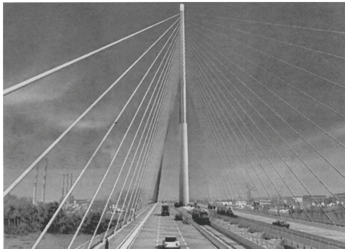
Figure 5: Model of designed bridge over river Sava at Ada Ciganlija in Belgrade
