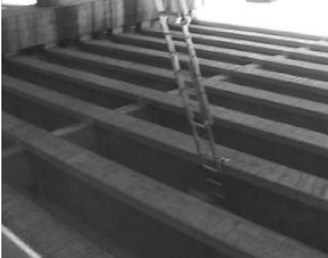
Figure 14: The lower deck of the bridge, possible location for displacement measurement
